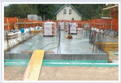
The layer of thermal insulation should be promptly protected from strong sunshine. Prior to installing reinforcement rods, seal off any potential gaps at the board joints or alongside the formwork with polyurethane foam or suitable adhesive tape in order to prevent any cement from leaking in while laying concrete. No sealing foil can be used when using SEISMIC boards. Next is the installation of reinforcement rods with spacers on top of the SEISMIC thermal insulation and concreting.
